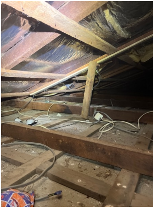
Image of pitch, roof frame and sarking
