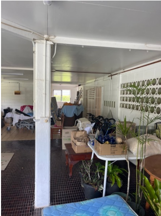
Image of floor coverings, heavy stored goods and equipment in the attached garage and laundry in the subfloor area
