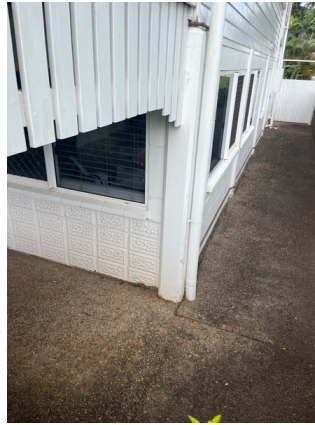
Image of no slab edge exposure
